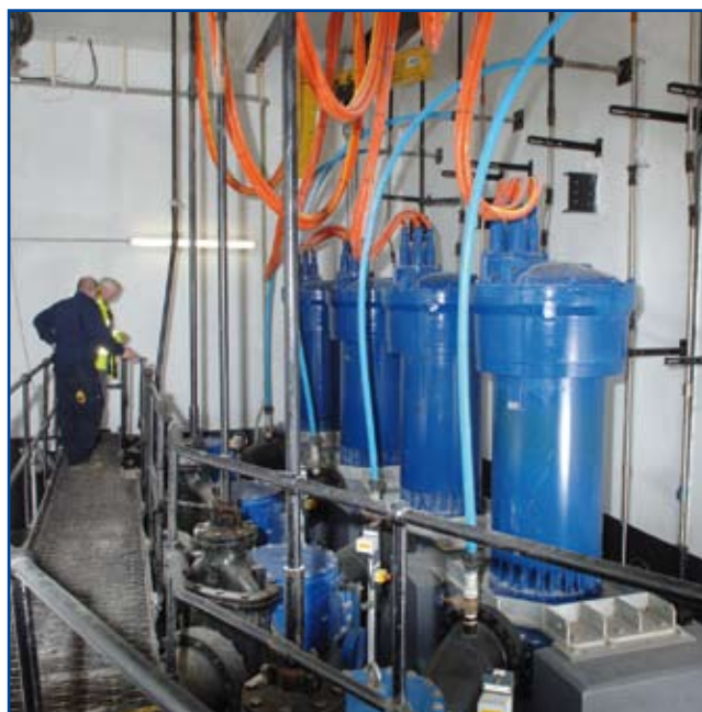
A typical flywheel installation, pumping raw sewage. 4 x Immersible pumps with 175KW motors and a duty of 300l/s at 35m head per pump.
